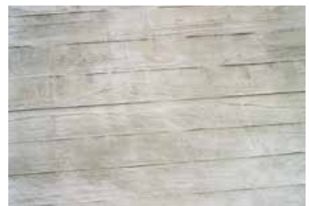
Board formwork texture reproduced in repaired areas
