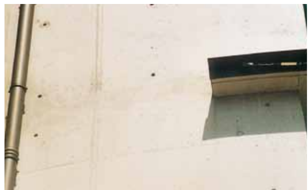
Filled areas largely toned down with KEIM Concretal-Lasur
