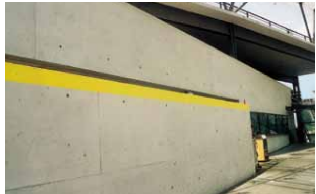
Uniform mineral surface with KEIM Concretal-Lasur
