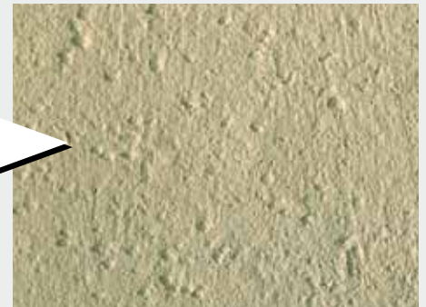
Intermediate or final coating with KEIM Granital
