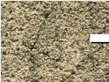
Existing render with cracks
